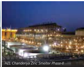
HZL Chanderiya Zinc Smelter Phase-II
